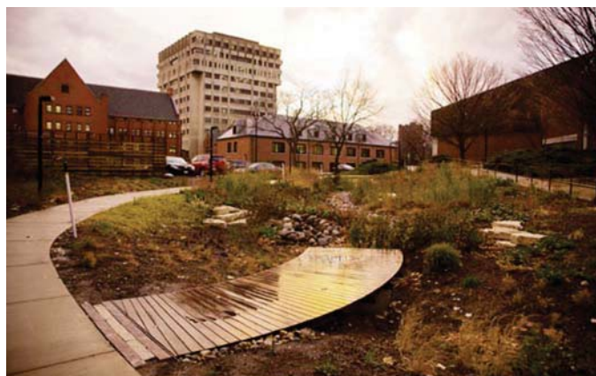
EXAMPLE OF A STORMWATER TREATMENT TRAIN
