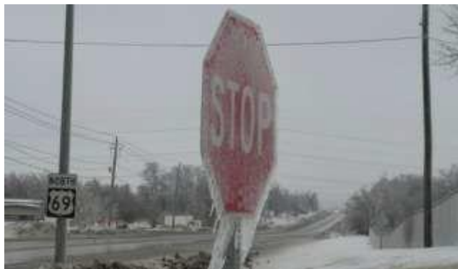
Figure 3.110. Ice on Stop Sign in Polk County, IA
