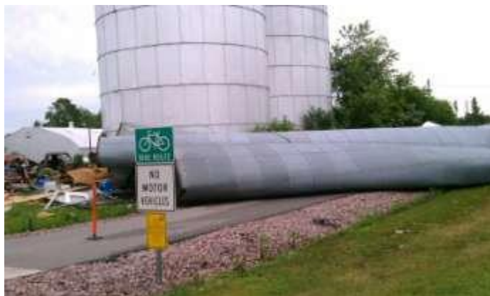
Figure 3.98. Severe Thunderstorm Caused Grain Bin Collapse, July 11, 2011
