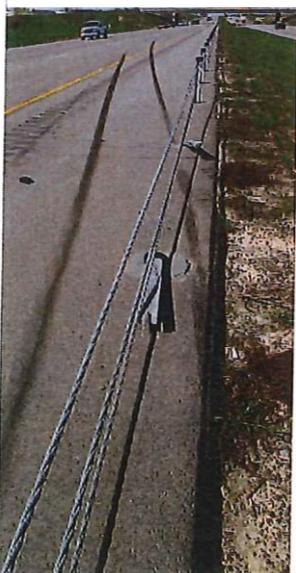
Although several different high-tension cable barrier types exist, they all use the same cable that consists of 3/8-inch-diameter galvanized steel cable with 3-by-7 construction (21 wires).
