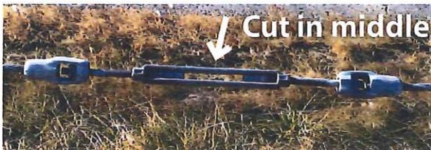
Always cut in the middle of the turnbuckle. Make the cut several hundred feet from the vehicle, midway between two undamaged posts where the cables are parallel and not being subjected to multiple forces.
