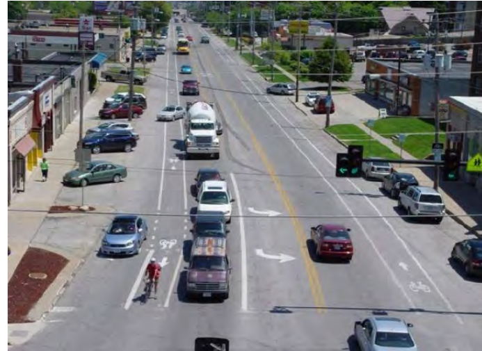
Road diets like this one on Ingersoll Avenue would not be viewed favorably.
